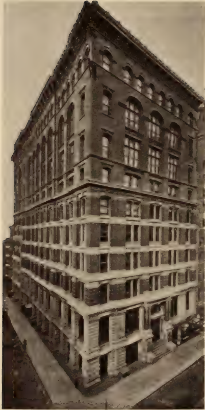
WESTERN UNION BUILDING.
